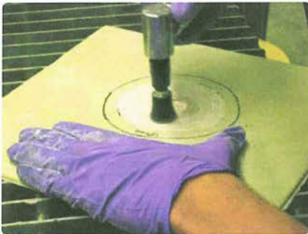
Figure 3-60. Taper sanding of repair area.
