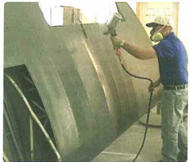
Figure 3-163. Applying a primer with UV blocking by spraying cross coats.
